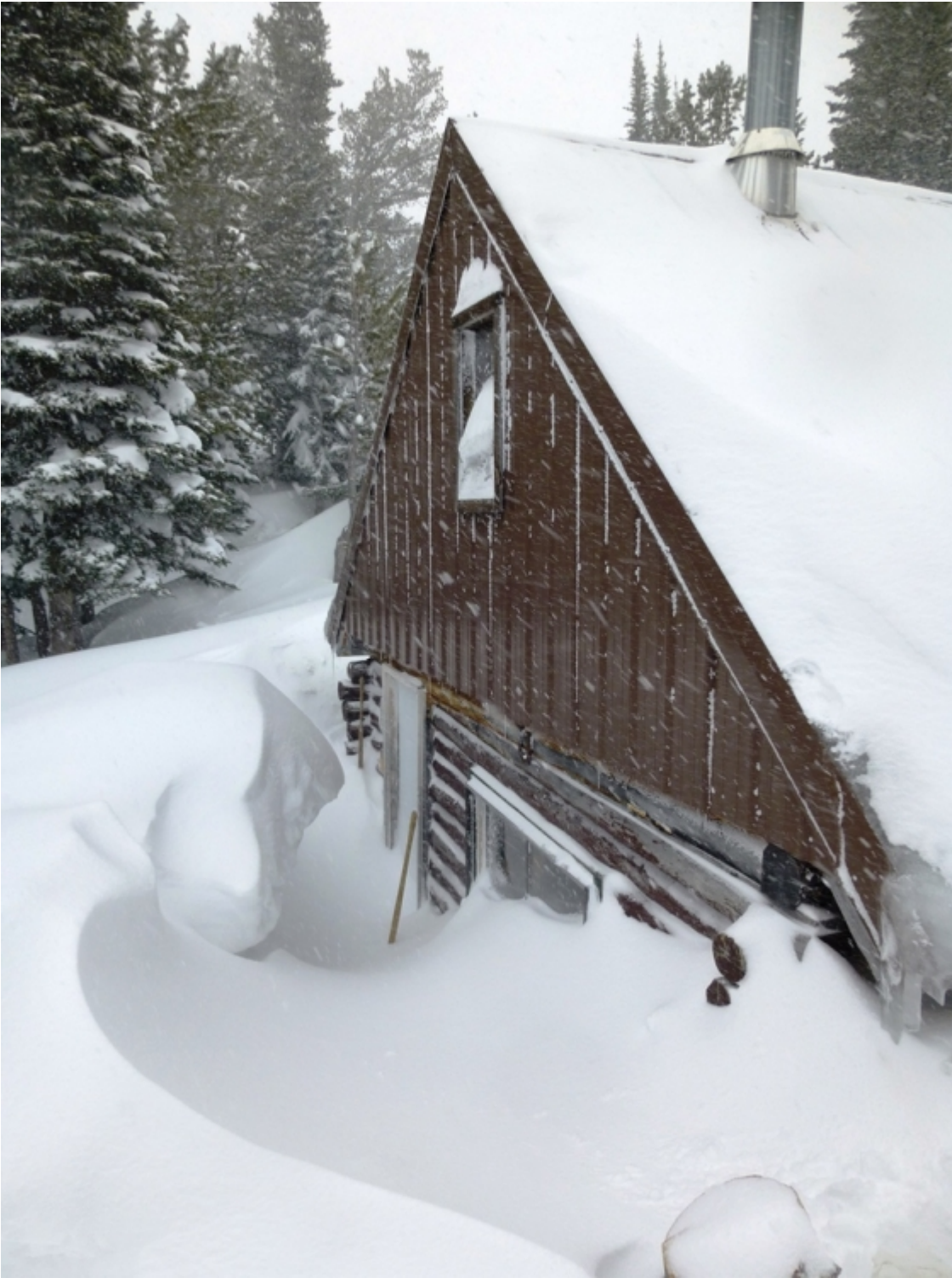
A cornice at the front door of the Round Lake Warming Hut is a sure sign that it's been snowing and blowing a ton, hence the Avalanche Warning! Photo: GNFAAC
